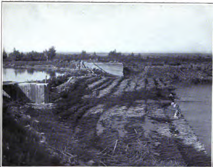
OLD DIVERSION DAM IN MILK RIVER, MONTANA. Temporary construction by community of farmers, with expensive brush and stone repairs.
